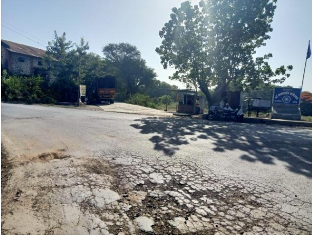
Existing Road Condition
