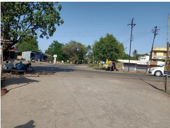
Existing Electrical Poles & Wires
