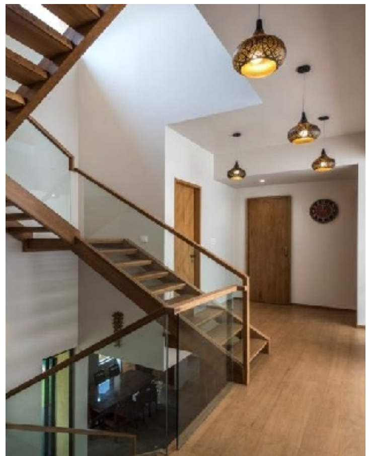
RIGHT Centrally located staircase divides public, semi-public and private zones acts as a central spine of house to make it lighter , veneer is cladded on M.S. structural skeleton. Chamfered wooden nosing of steps gives semi transparent character, glass railing with wooden handrail and thin wooden bridge gives proper visual connectivity.
