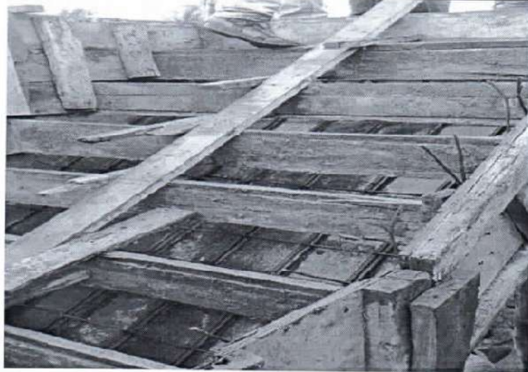
Staircase Reinforcement
