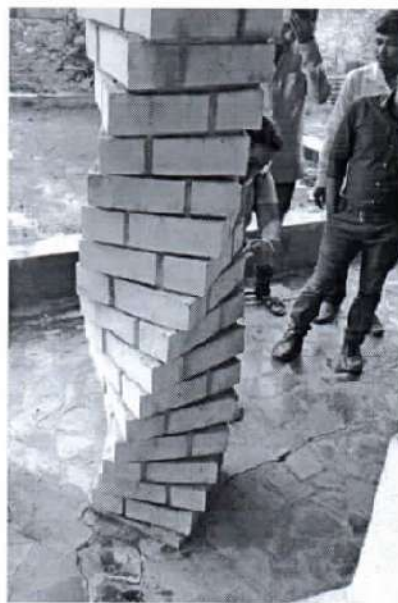
Twisted Pillar in Flemish Bond
