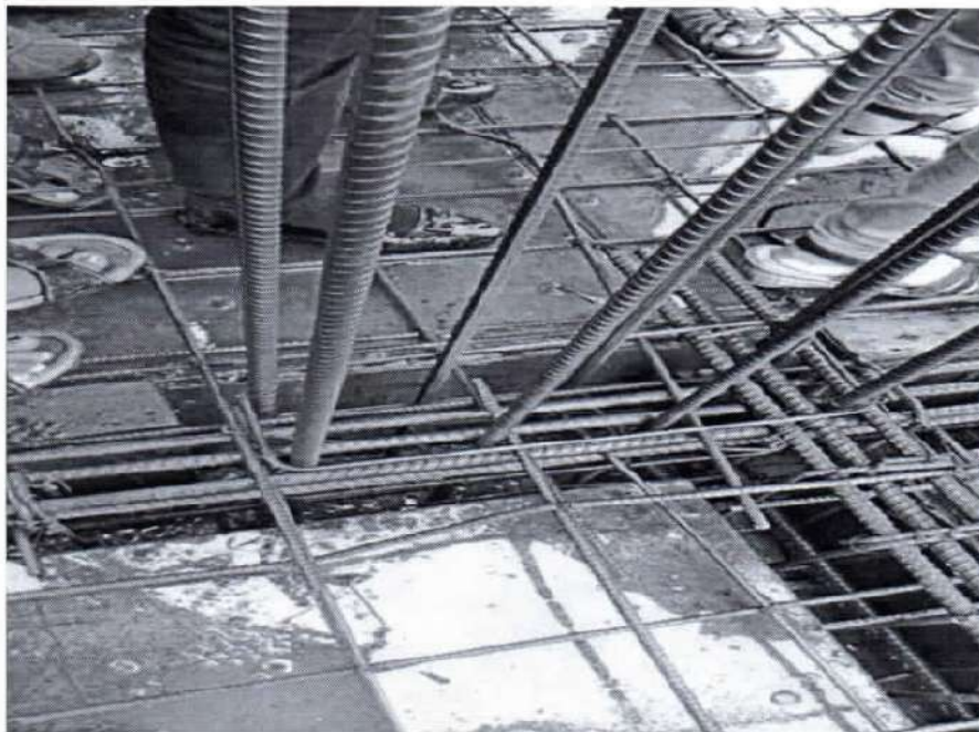
Reinforcement at Beam & Column Junction
