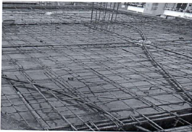
Two Way Slab Reinforcement
