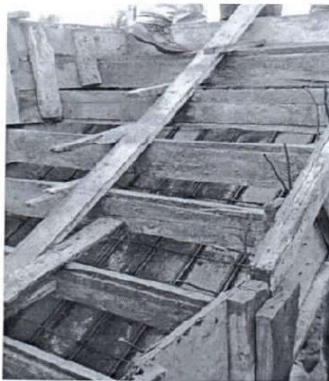
Staircase Reinforcement
