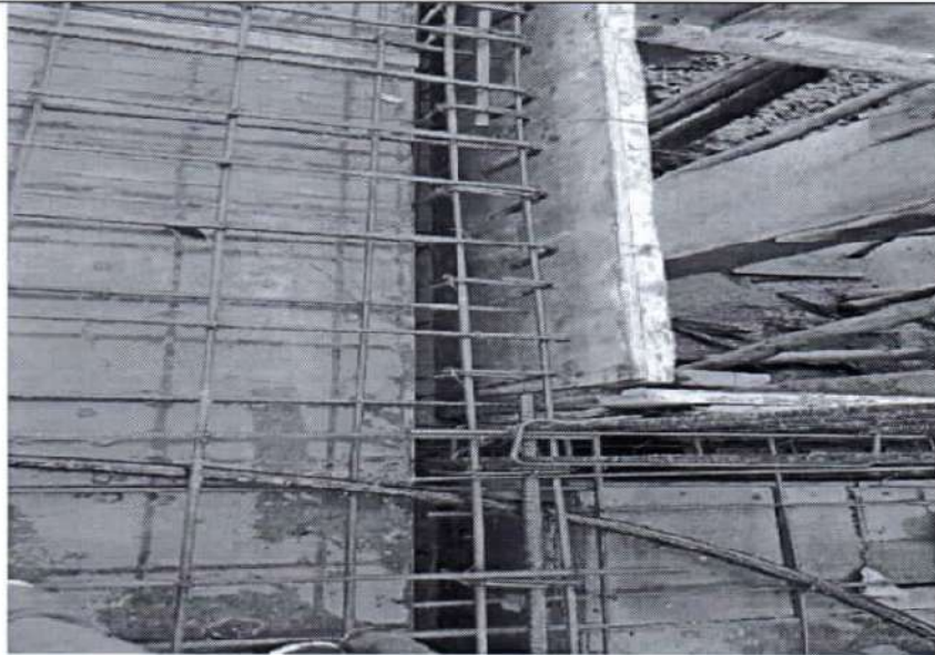
Reinforcement at Beam Junction
