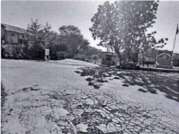
Existing Road Condition
