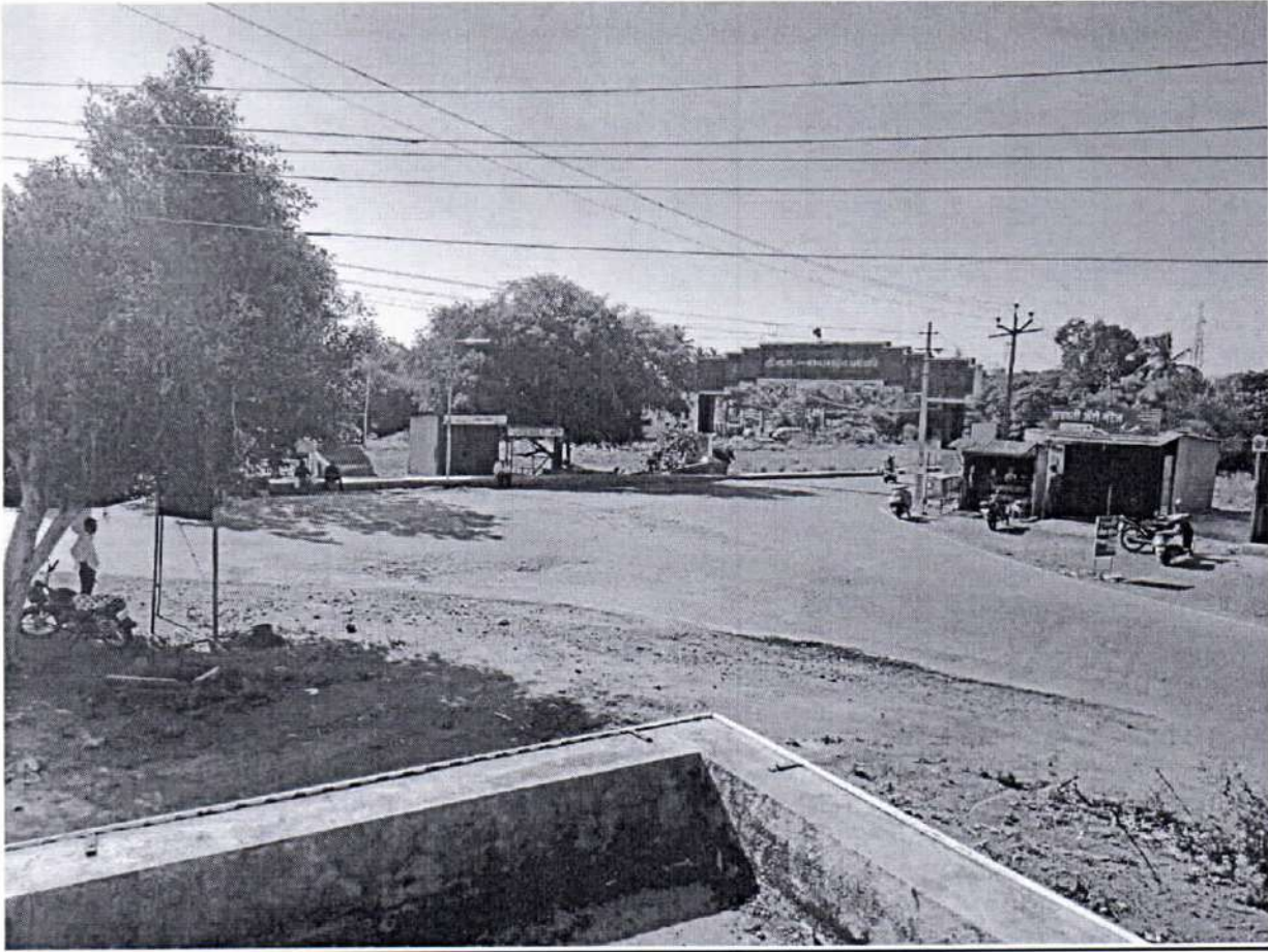
Existing condition of chowk
